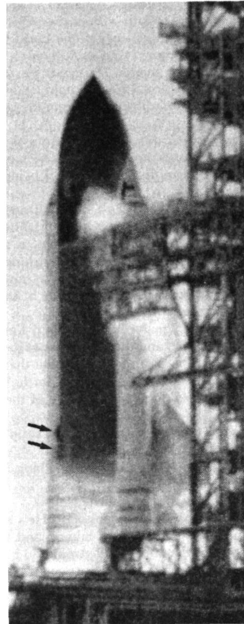
**FIGURE 14.** Puffs of black "smoke" (fine, unburned particles) were seen escaping from the same place where the flame was observed.
